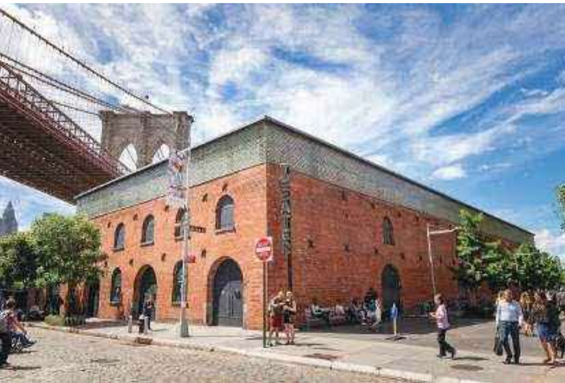
St Ann's Warehouse in New York City transformed a former tobacco warehouse into a performing arts venue with the addition of a new steel structural frame and a glass brick clerestory, prolonging the lifespan of the warehouse.
